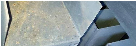
Fractionator redistributor after decontamination
